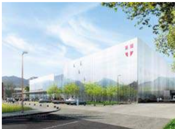
Hospital Chambéry - Chambéry (France)
